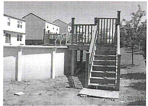
Figure 8. Gate at top of stairs. Safety barrier measurement for the gate (48 inches minimum height) is taken from the last stair if gate is flush with edge of deck floor or is taken from the floor if gate is not flush with edge.
